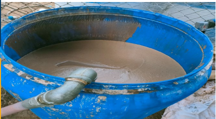
Field mixing of HYPER-ER weighted slurry
